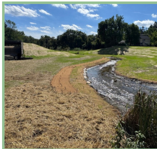
NEW CHANNEL FLOWING AROUND FORMER DAM
