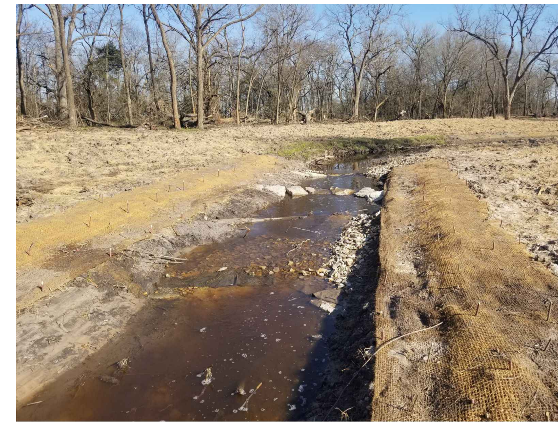
BOULDER CONSTRUCTED RIFFLE CONSTRUCTED MARCH 2019
