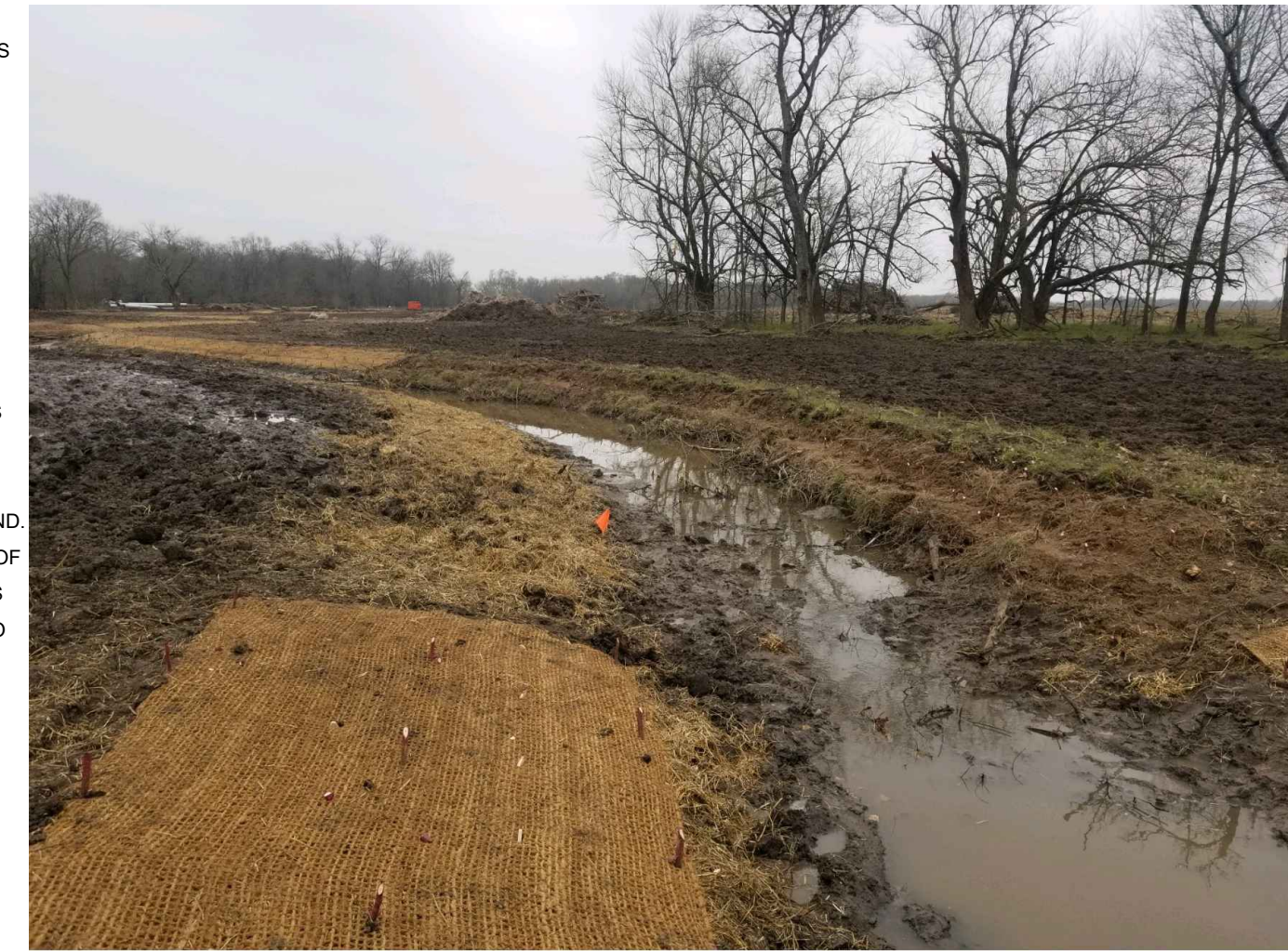
TOE WOOD WITH COIR SOIL LIFTS CONSTRUCTED
