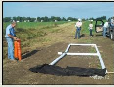
One of our farmer leaders explains how this blind inlet works to reduce sediment and nutrient loss into tile drains.
